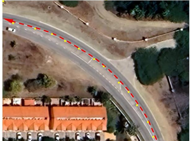
Widing Section # 3 (Roundabout Marriott Hotel, Bakval, Noord)
