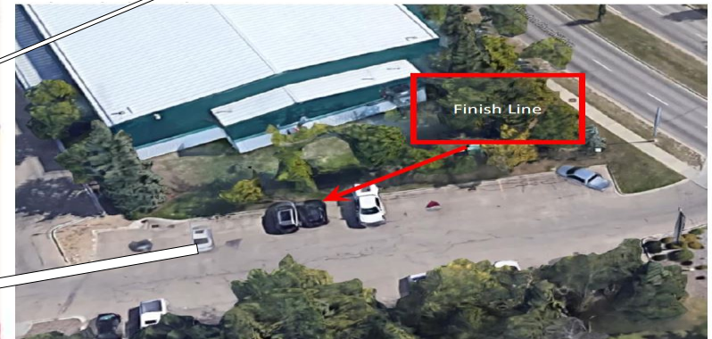
Finish line is a yellow parking stall line next to a crack in the curb, in line with the back door of the curling club. (Parked vehicle in photo blocks the view)
